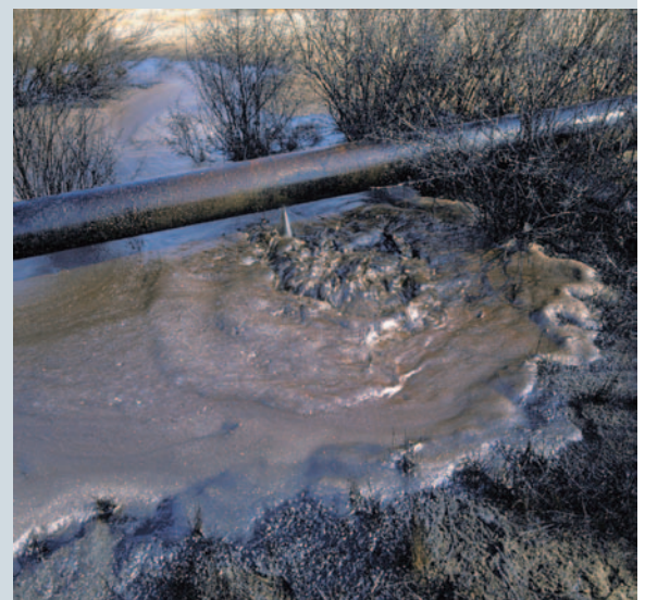
FIGURE 2: Oil leaking from a pipeline (Source: Russ Widstrand/Workbook Stock/Getty Images)
